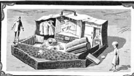
STORM DAMAGE TO HOUSE: REPAIRS- $1200
